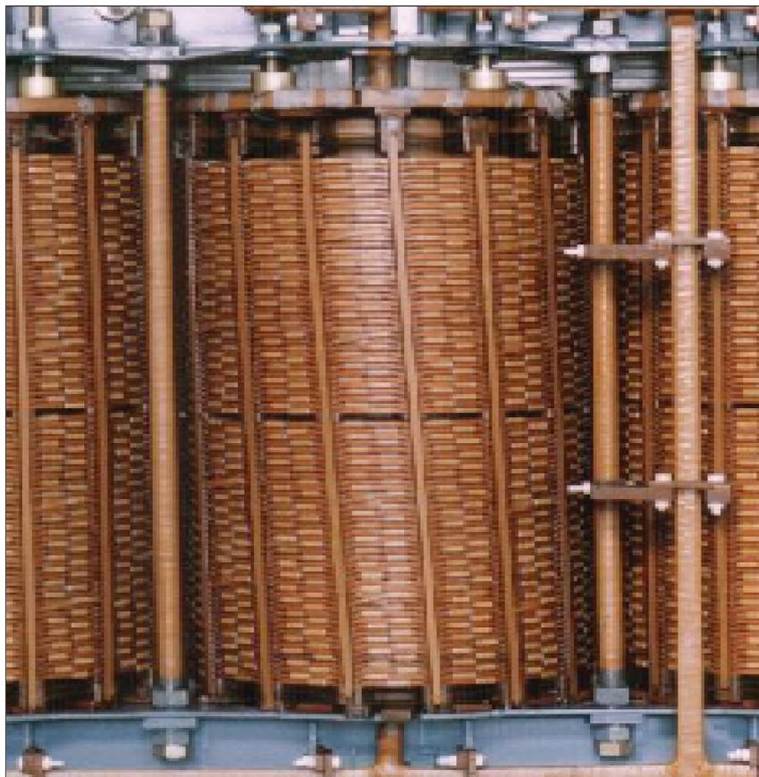
P-1. 5 MVA, 33/11.55 kV TRANSFORMER
