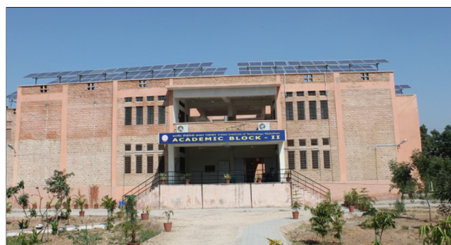
FIG. 1 ACADEMIC BLOCK II BUILDING, LOCATED AT 'IIT JODHPUR' JODHPUR.
