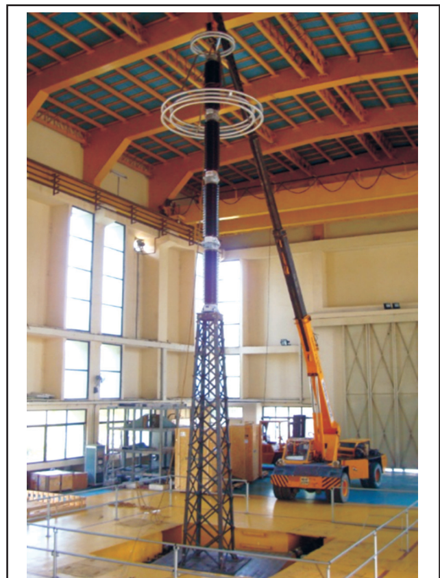
FIG.1 624KV-20MASURGE ARRESTER MOUNTED ON SHAKE TABLE.
