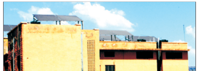
FIG. 2 ACADEMIC BLOCK I BUILDING, LOCATED AT "IIT, JODHPUR" JODHPUR
