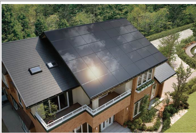
FIG. 1 (A) TYPICAL BIPV INSTALLATION IN RESIDENTIAL BUILDINGS
