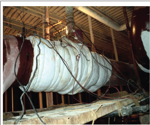
FIG. 10 IMAGE OF IN-SITU HEAT TREATMENT OF ATTEMPERATOR (LHS)
