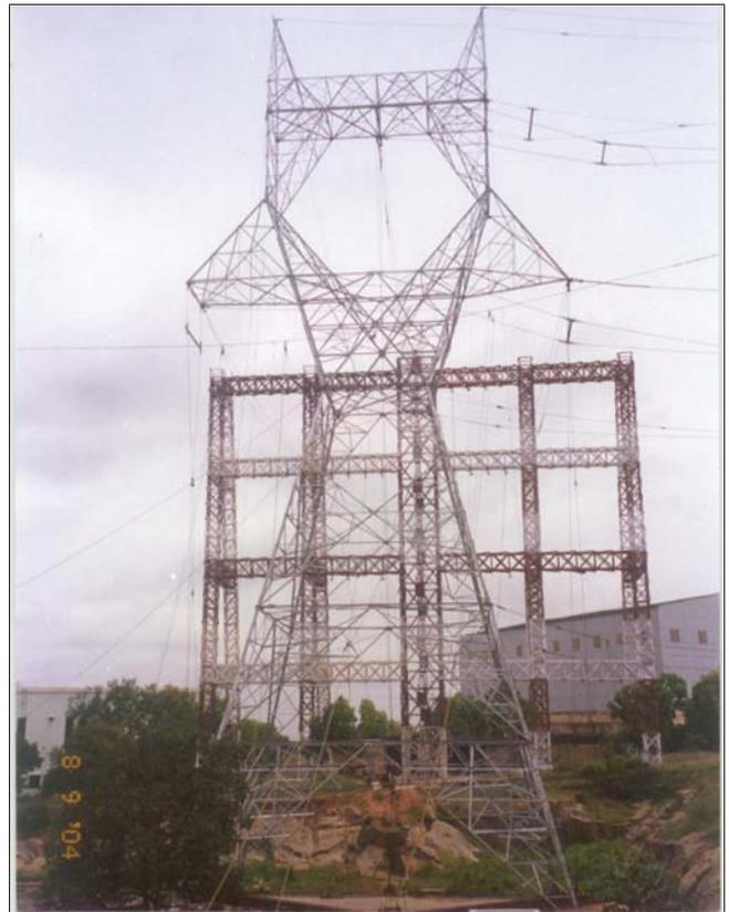
FIG. 7 TOWER WITH RIGGING ARRANGEMENT
