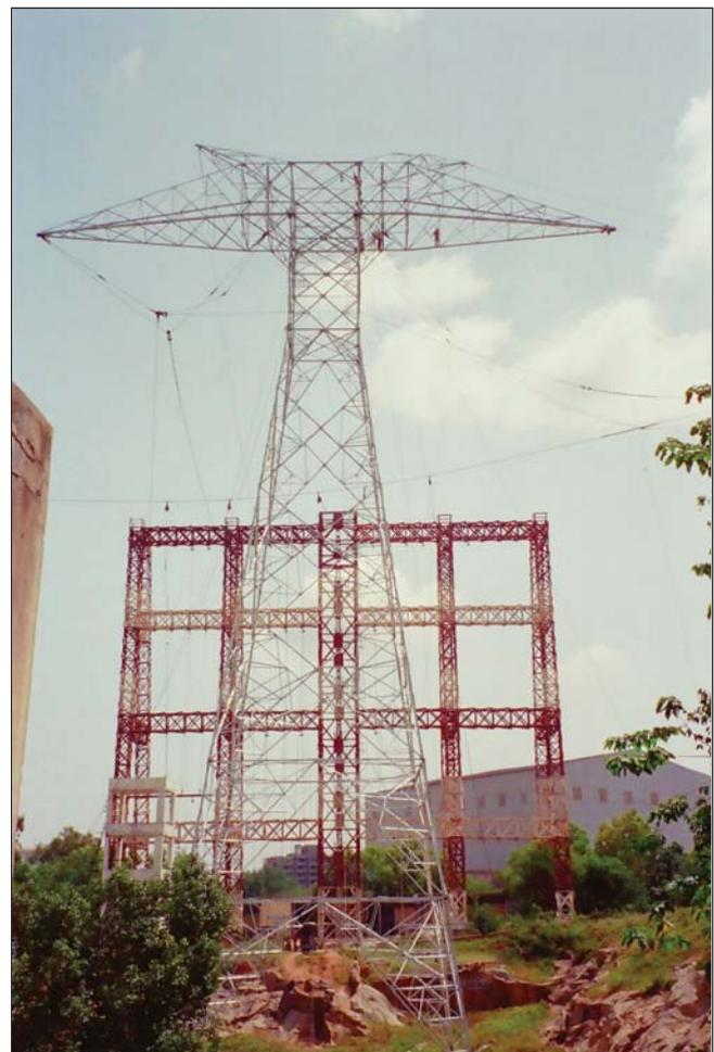
FIG. 4 800 kV HVDC 'Y' STRING TOWER
