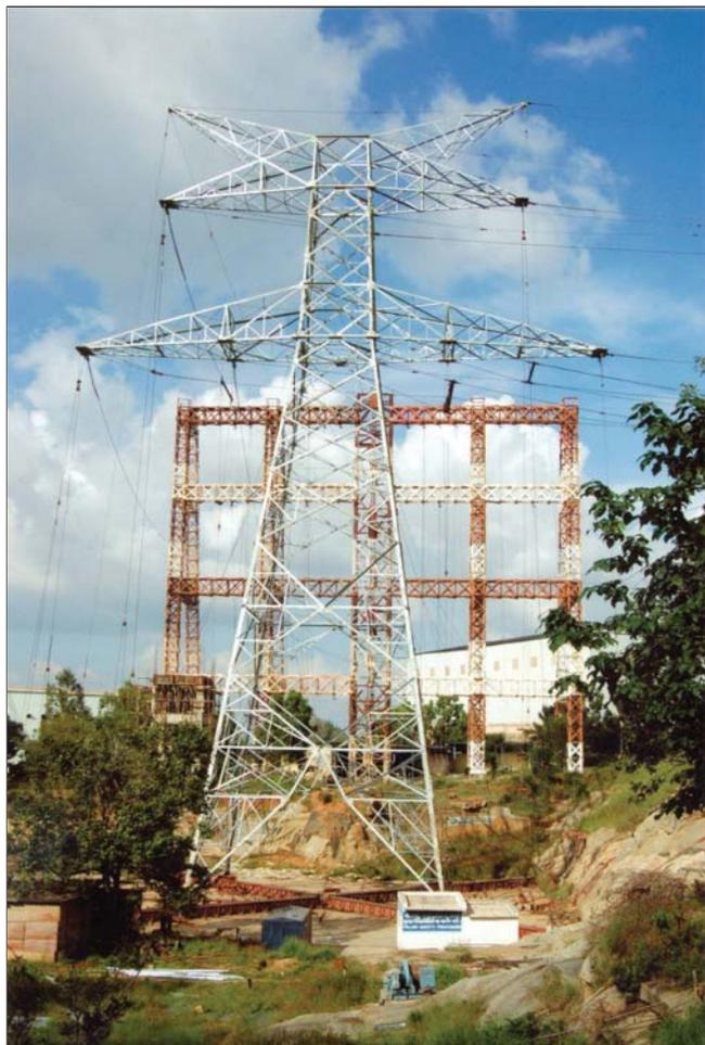
FIG. 5 400 kV D/C TYPE 'SET-70' TOWER
