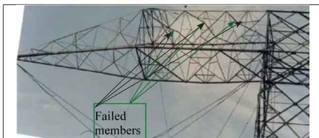
FIG. 9 CROSSARM (N TYPE) FAILURE AT TOP PLAN
