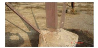
**Figure 4.** Snapping of stub angle.
