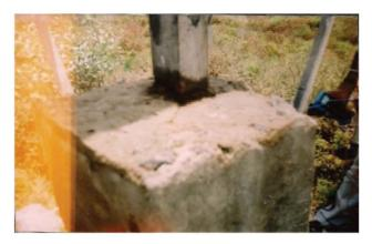
Figure 1. Formation of pitting corrosion at the angle concrete interface
