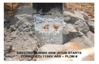
Figure 2. Disintegration of constituent materials of coping concrete.
