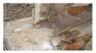
Figure 3. Bulging of Stub angle.
