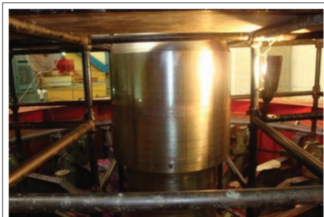
FIG. 4. PATCHING MADE ON 914 MM DIAMETER REGION OF ROTOR SHAFT FOR PAUT
