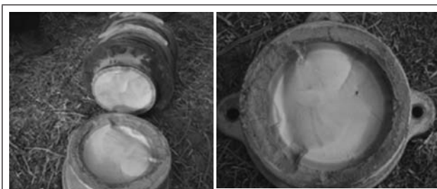
FIG.1. A TYPICAL VISUAL INSPECTION OF FRACTURED PORCELAIN POST INSULATOR
