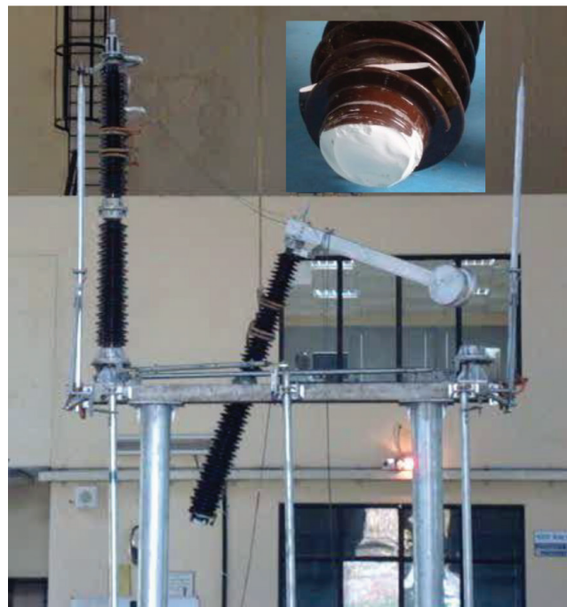
Figure 9. Disconnector post insulator shear.
