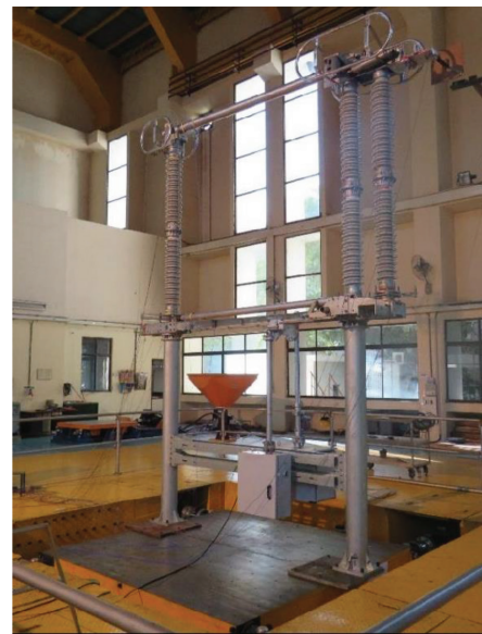
Figure 1. 245 kv disconnector mounted on tri-axial shaker system: Disconnector closed and ground switch open.
