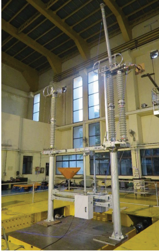
Figure 2. 245 kv disconnector mounted on tri-axial shaker system: Disconnector open and ground switch closed.
