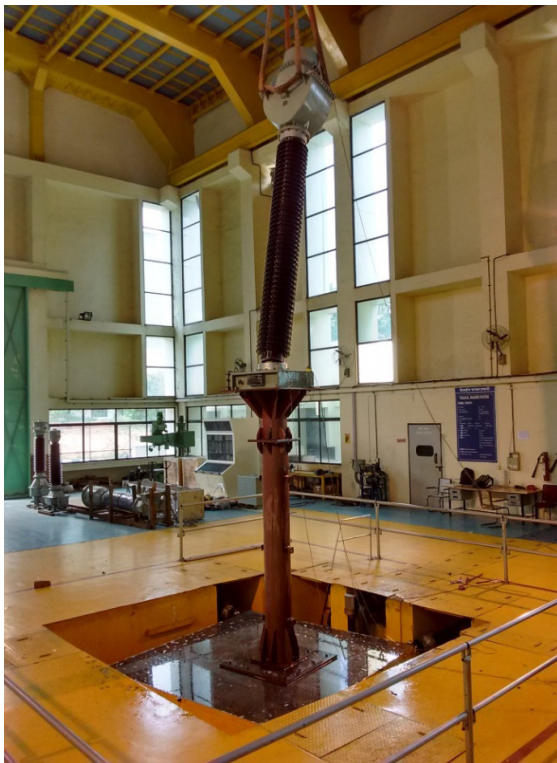
Figure 3. Live tank current transformer on shake table after failure.
