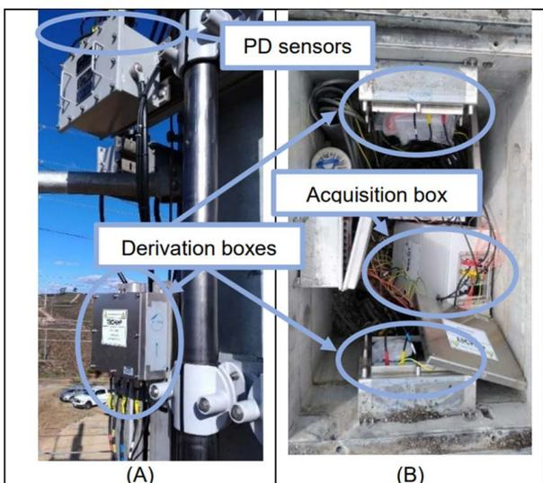
**Figure 10.** Installation of the measuring system (A) On the outdoor terminations and (B) In the joint bays.
