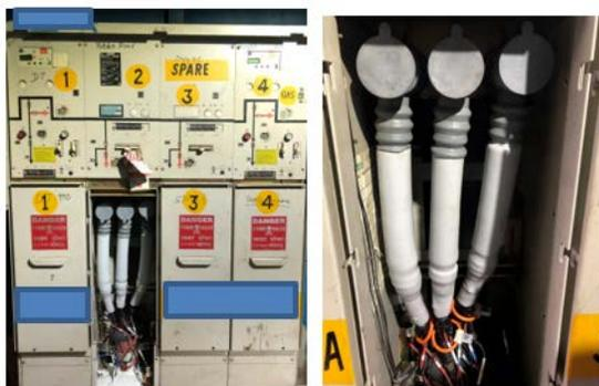
**Figure 3.** Field installation of cable terminations with voltage and current sensors.
