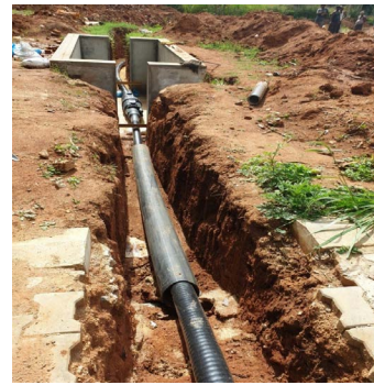
Figures 8 and 9. Cable laid through HDPE pipe under soil and cable laid in open tunnel with fixed conditions.
