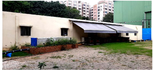
Figure 7. Cable laid in air through closed tunnel.
