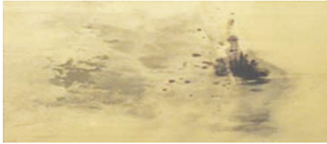
ARC – INSIDE TANK DUE TO INTER TURN FAULT
